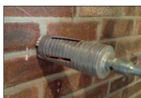
1. SELECT A 65MM CORE DRILL.
